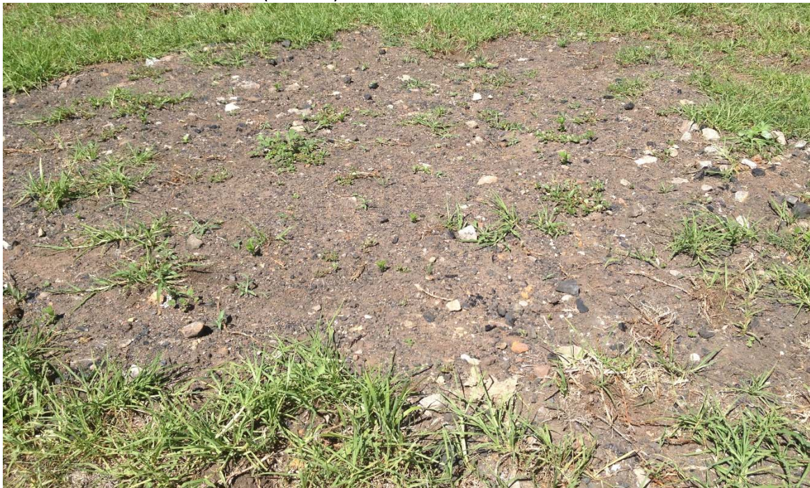
Photo 5: Example of visible fill material.
